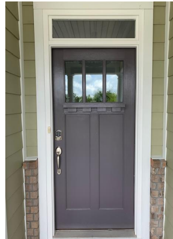
Upgraded Front Door Style with 3 windows
