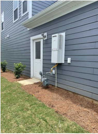
Standard Tankless Water Heater mounted outside Or Upgrade and move to garage interior
