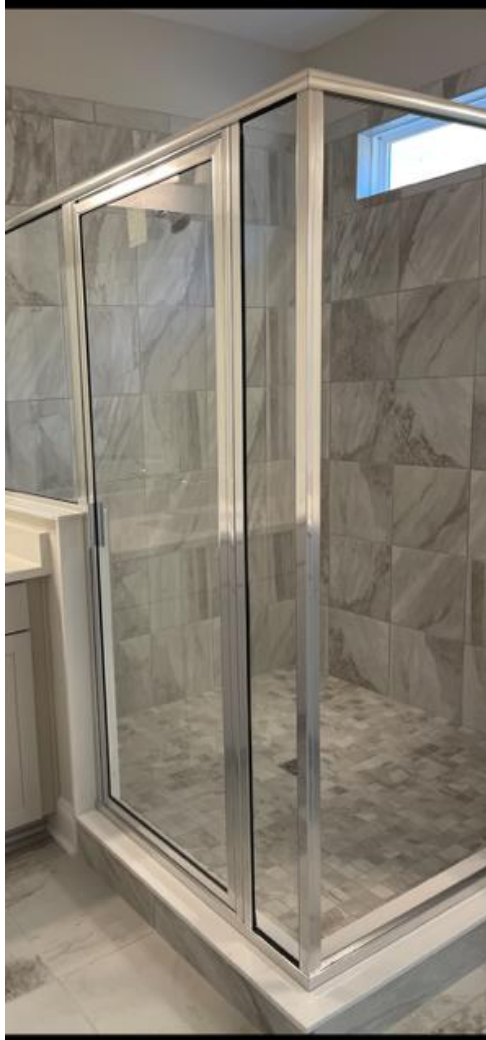
13x13 Tile Straight/Stacked Installation Owner's Bath Upgraded 2x2 Shower tile floor
