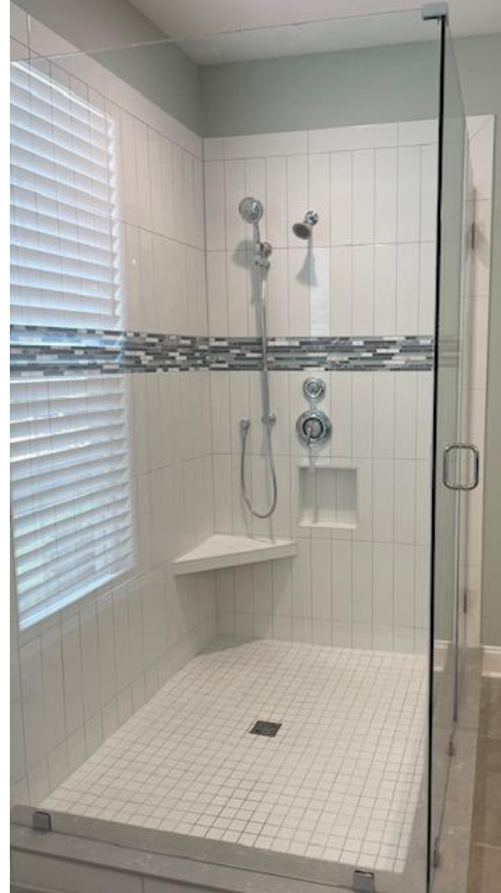
4x16 Subway Tile Vertical Stacked installation With 6" optional accent
