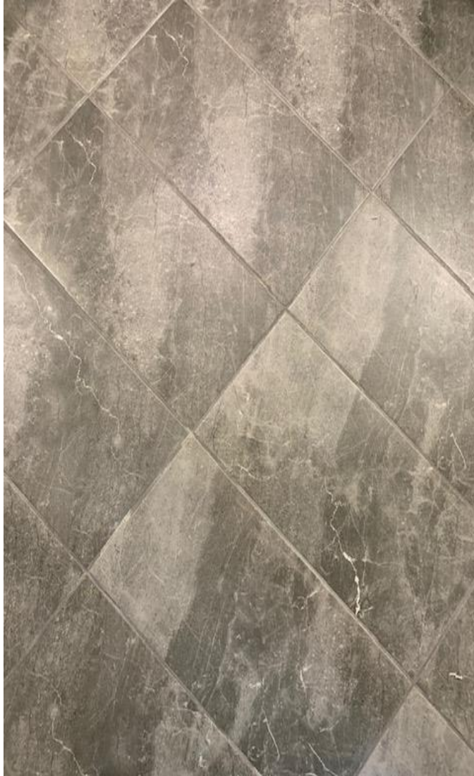
Bathroom floor 12x24 Tile Straight lay Installation
