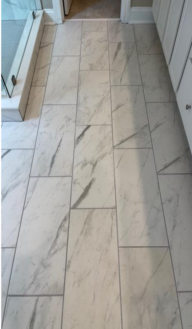
Bathroom floor 12x24 Tile Brick lay Installation
